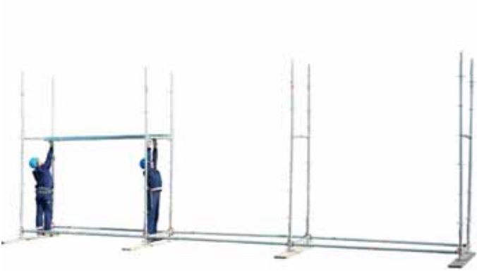
13 • erecting metal ledger planks
