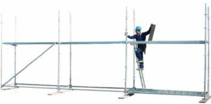
21 • passage to the upper level
