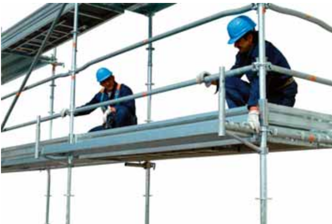
45 • inserting the wedge
