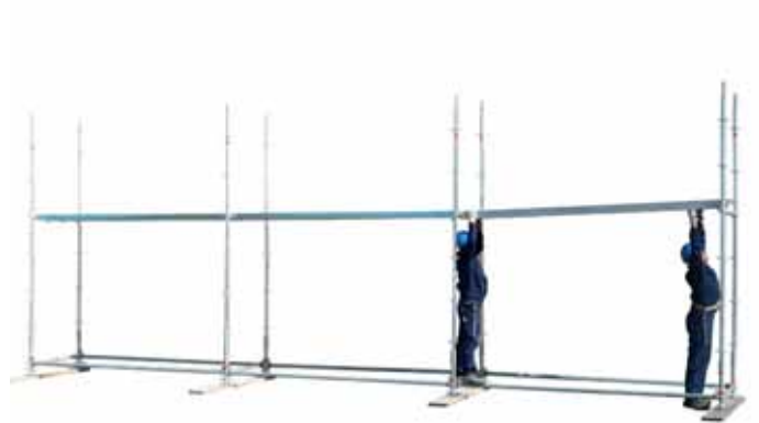
16 • erecting ledger board with trapdoor
