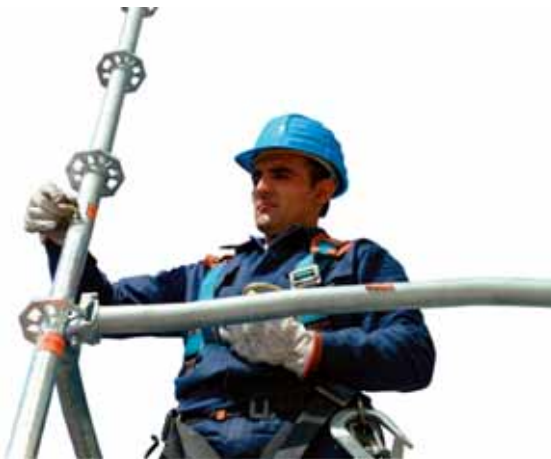
32 • inserting spigot pin connector
