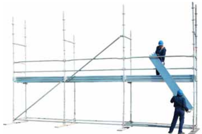
36 • erecting level 2 scaffolding
