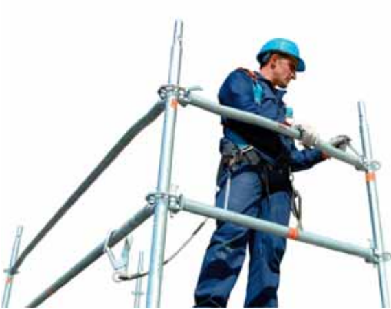
25 • erecting side fencing structure
