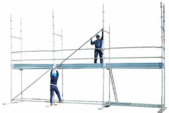
35 • erecting diagonals every 4 fields per floor
