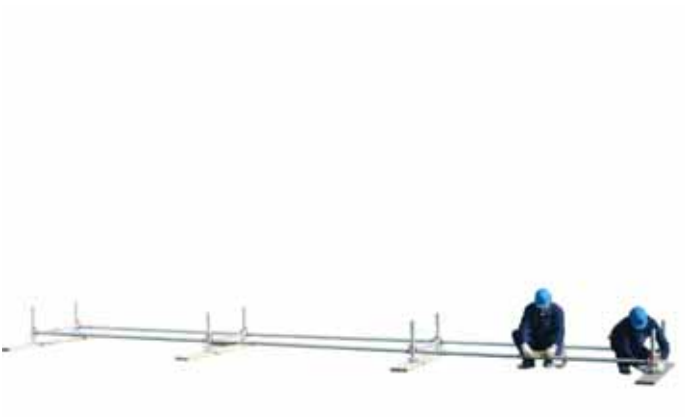
8 • checking the final level
