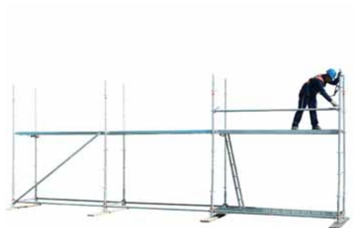
23 • erecting level 1 guard rail
