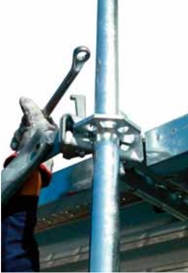
19 • erecting diagonals
