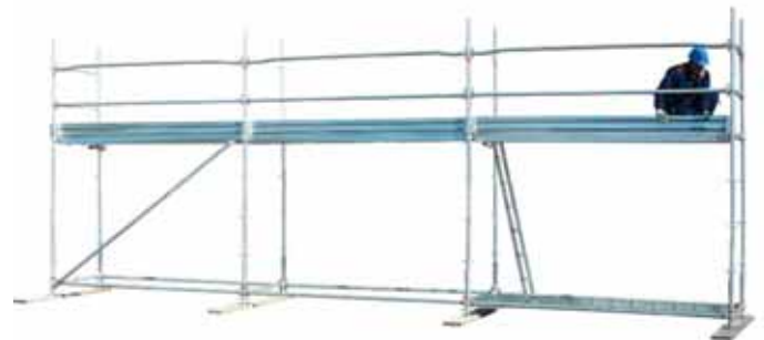
29 • erecting façade toeboard
