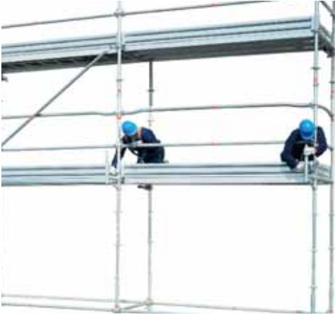
43 • erecting bracket
