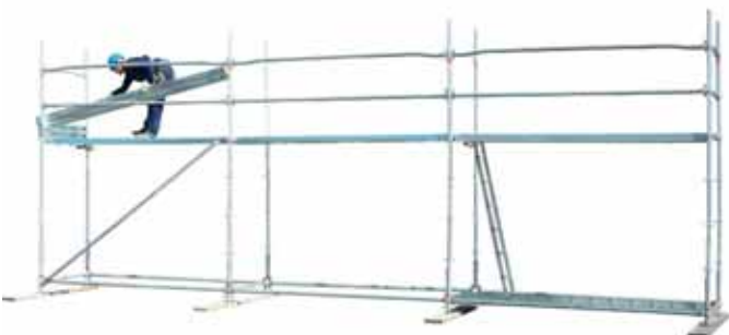
27 • erecting side fencing toeboard
