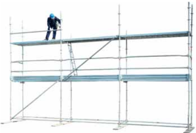
39 • erecting level 2 guard rails
