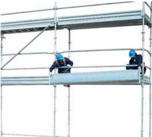
44 • erecting overhanging plank
