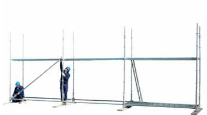
17 • erecting diagonals
