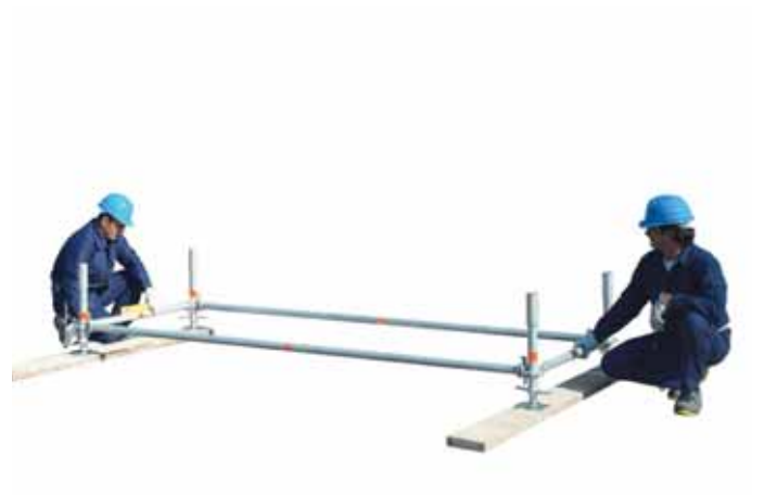
6 • levelling the transverse
