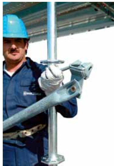
18 • erecting diagonals
