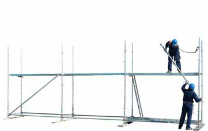
22 • erecting level 1 guard rail
