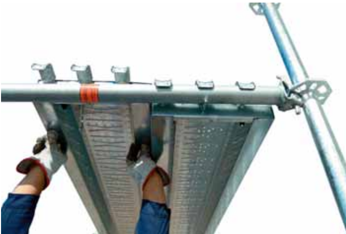
14 • erecting metal ledger planks
