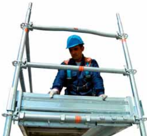
26 • erecting side fencing structure
