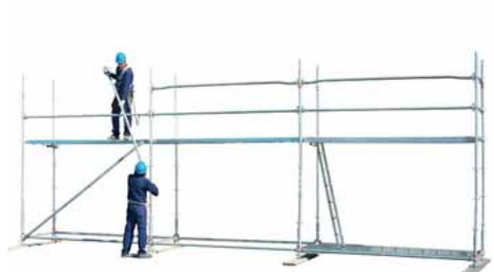
24 • erecting level 1 guard rail
