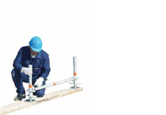
2 • levelling the base
