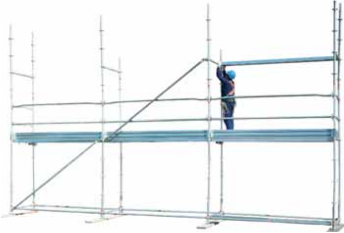
37 • erecting level 2 scaffolding
