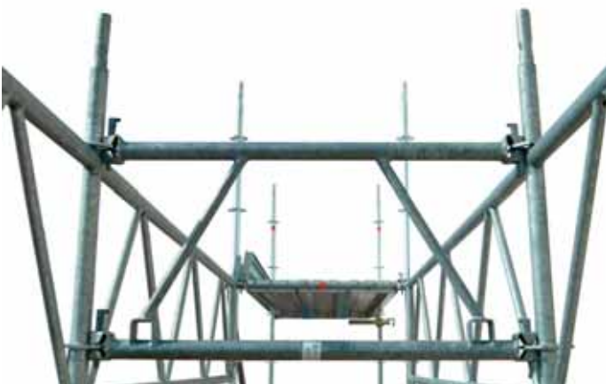
51 • erecting carriage beam couplings
