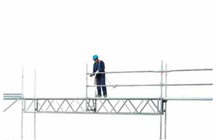
52 • erecting carriage beam guard rail
