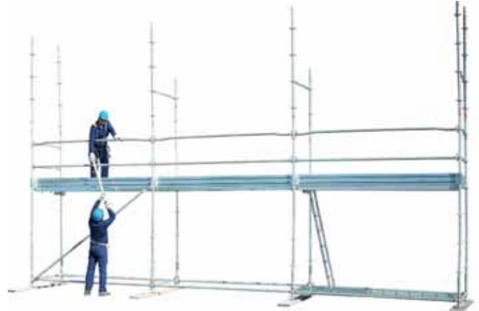
34 • erecting level 2 ledgers and guard rails
