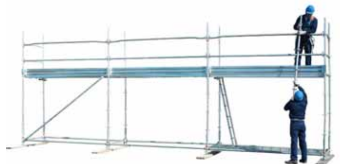
30 • erecting the upper uprights
