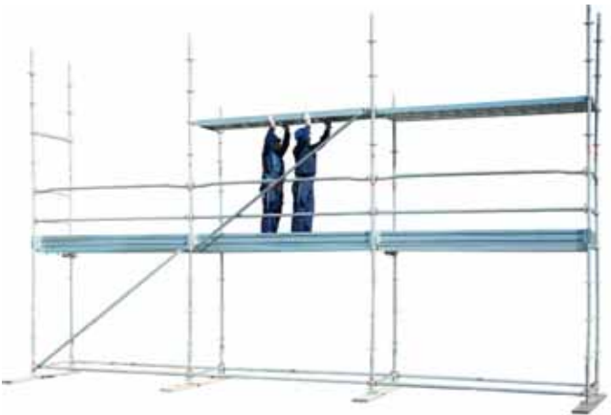
38 • erecting plank with trapdoor
