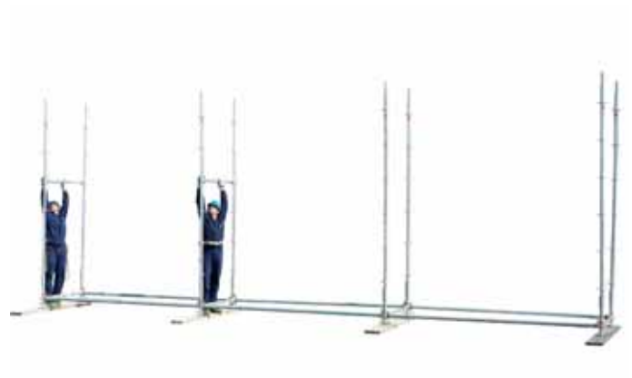
11 • erecting the upper ledgers
