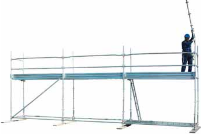
31 • erecting the upper uprights
