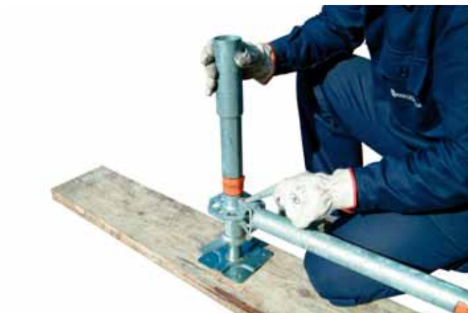
3 • ledger erection
